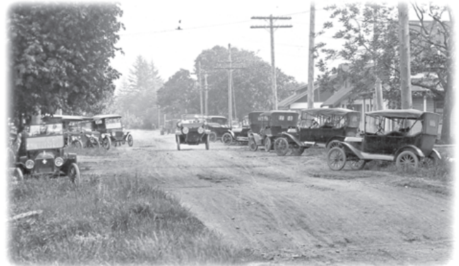
This would have been a good road in a typical Oregon town in the early 1920s. Of course in winter it would turn into deep mud that would have challenged the hardest motorcyclist. Rural roads wouldn't have been as highly developed or maintained. (And yes, that is a woman driving the car coming towards us.)
